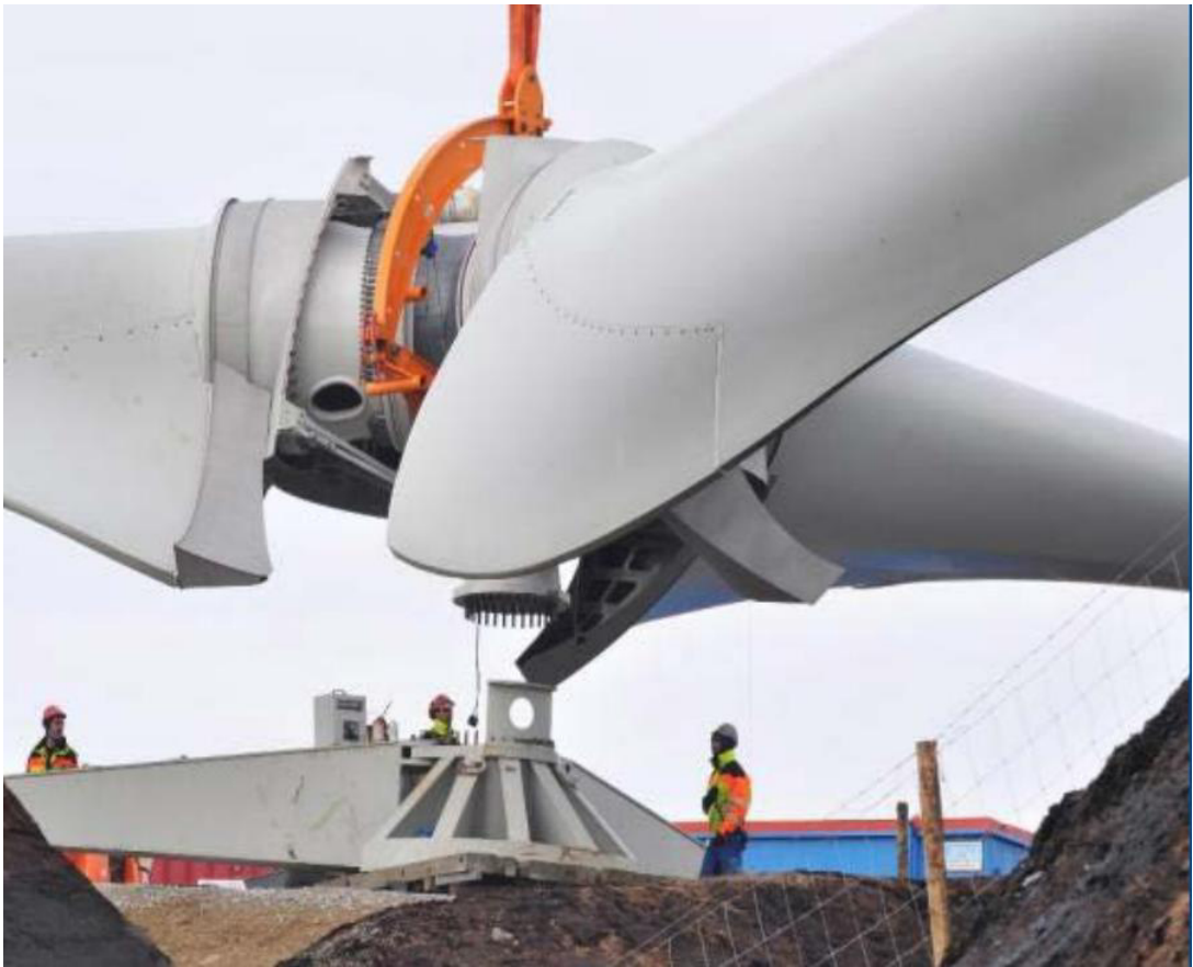
Plate 3.4: Assembly of wind turbine blades 2
